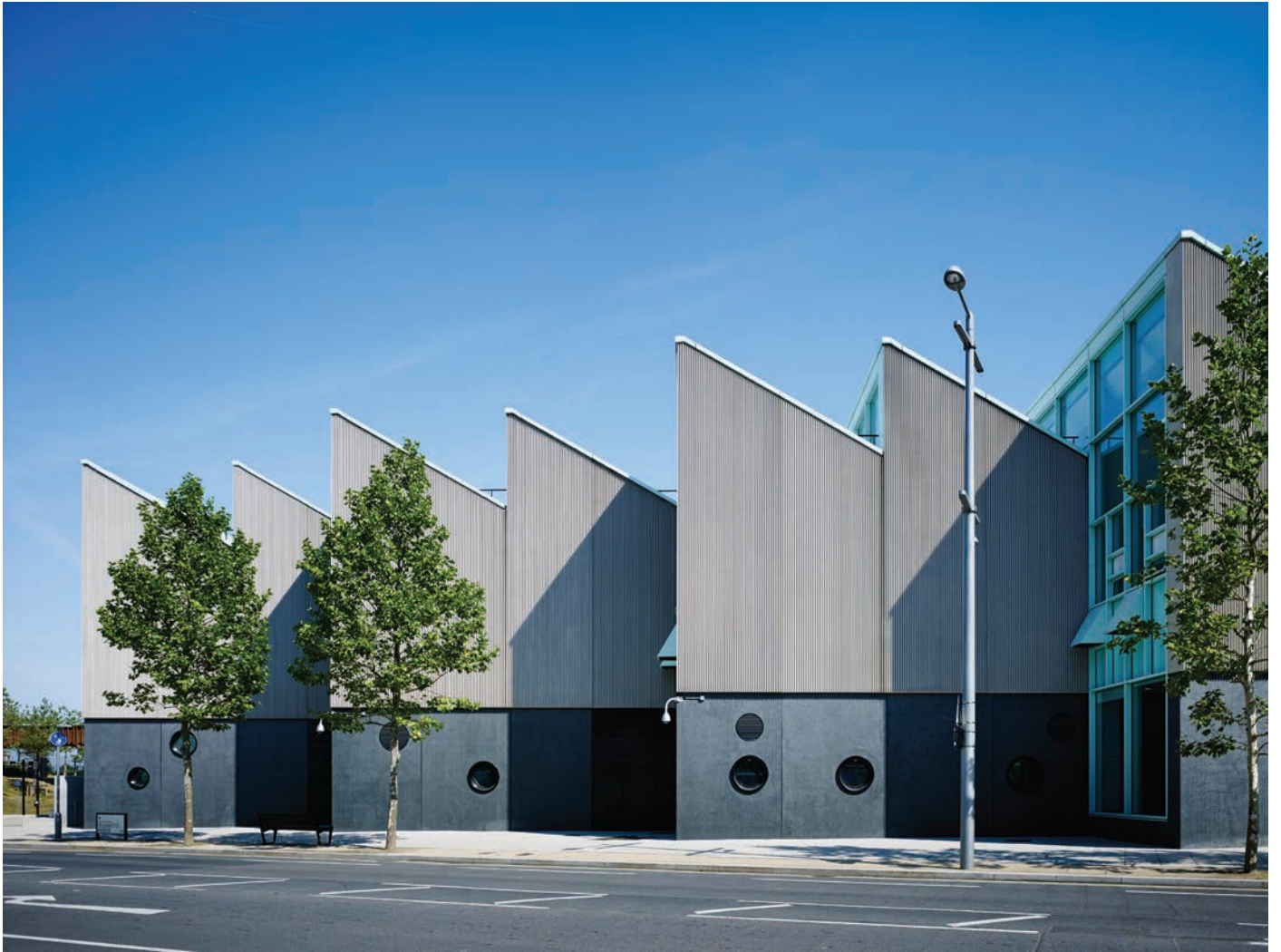
View of the Specialism Buildings dramatic saw-tooth roof
