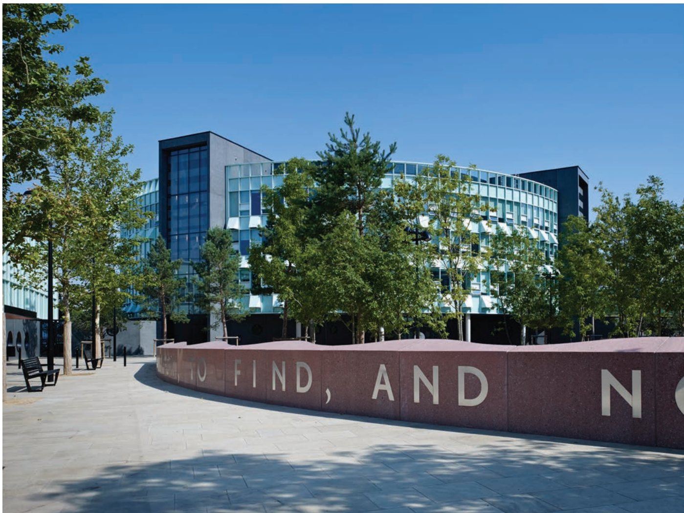
View of Chobham Academy from the playground
