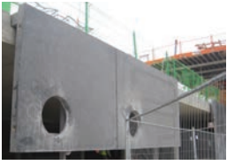
Concrete podium wall
