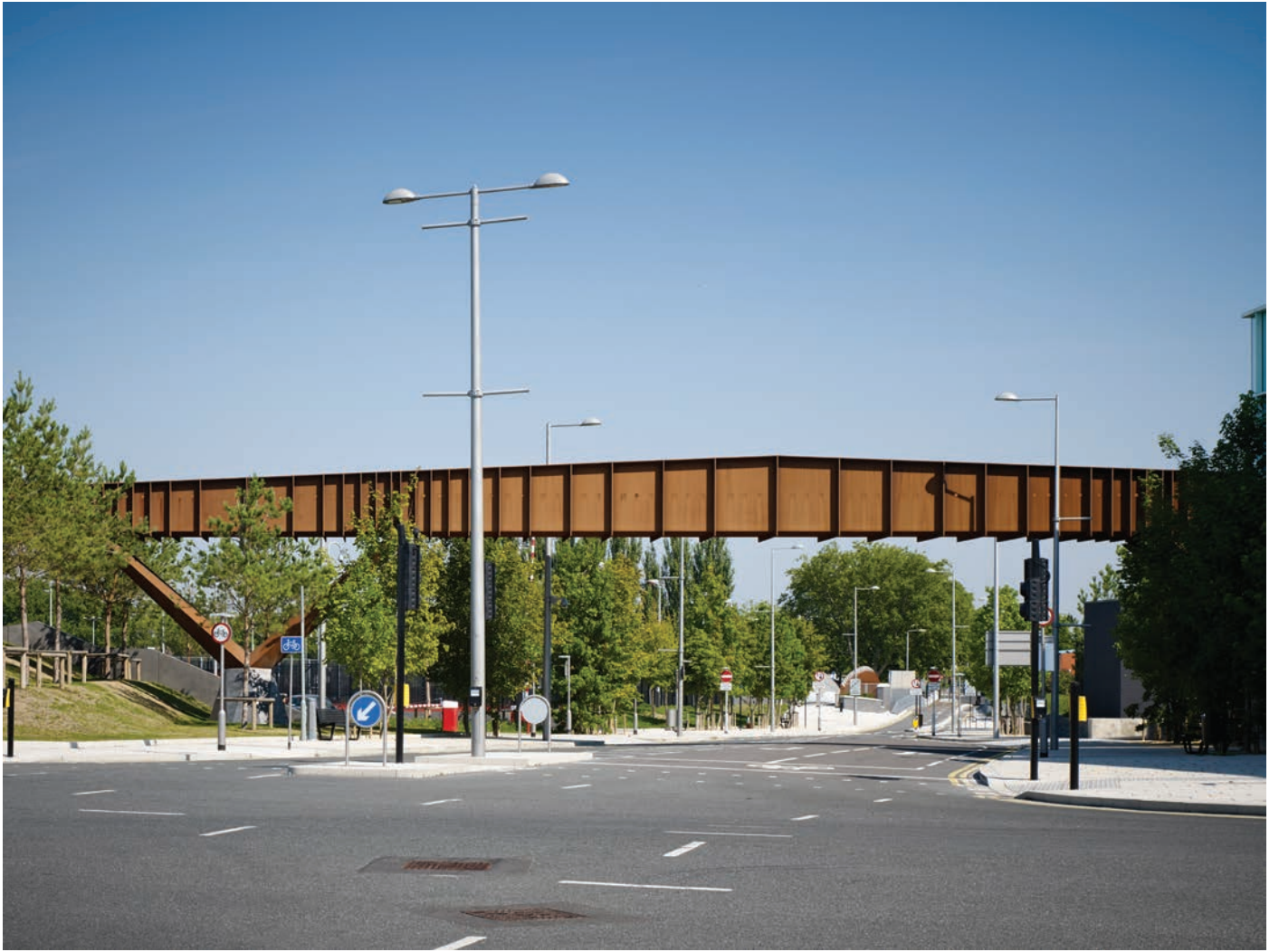
The 95-metre footbridge extends the school's reach over Temple Mill Lane
