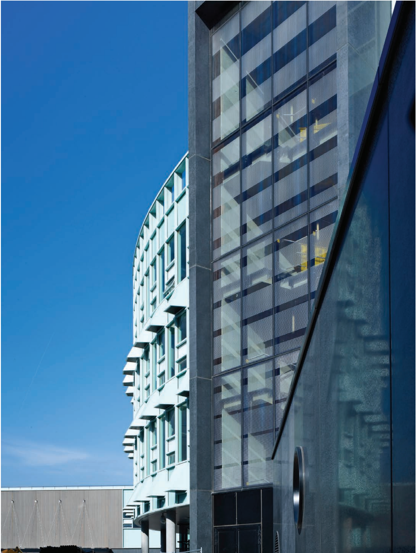
Main Building stair tower
