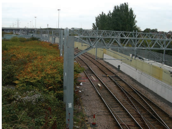
Stratford railway line running alongside the site
