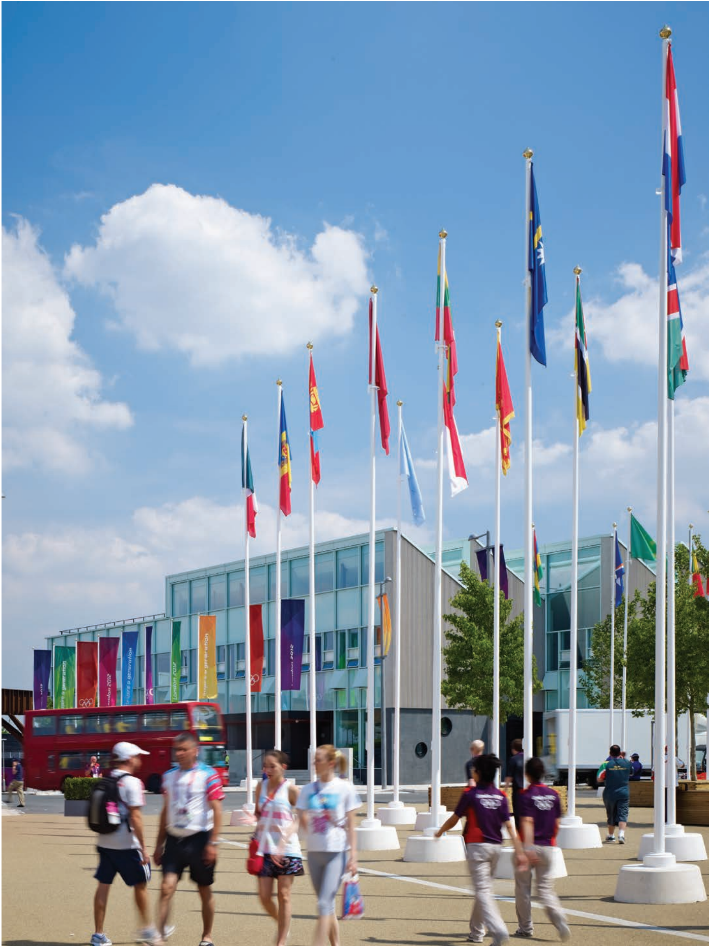
Approach to the Specialism Building during the Olympic Games
