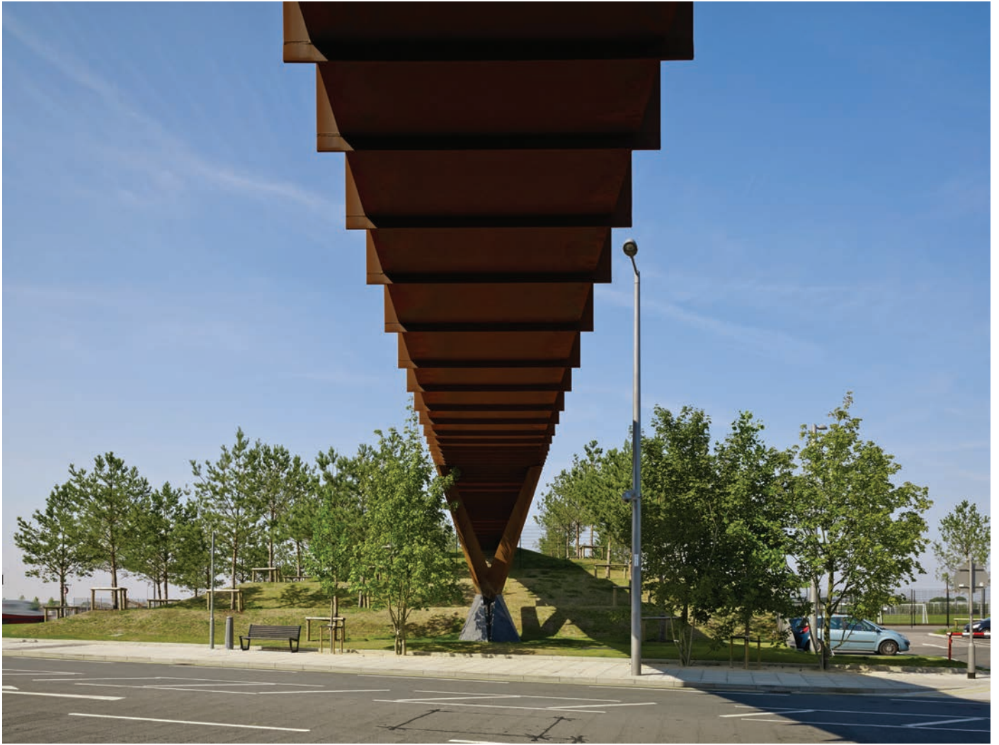
The 95-metre corten steel footbridge extending across to Temple Mill Lane
